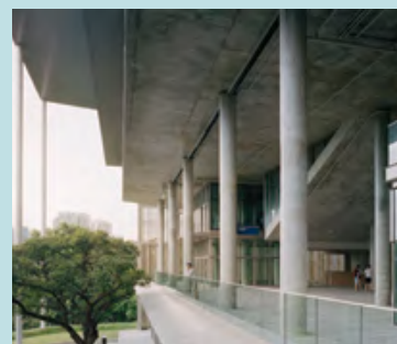
An exterior view of SDE4. Image: NUS College of Design and Engineering and Serie Architects / Rory Gardiner.
