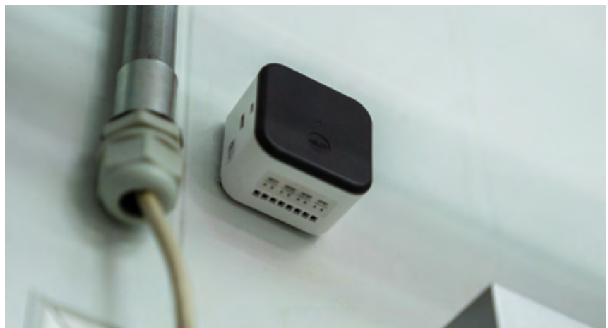
Relying on continuous power, the access controller is a small device that is optimally installed inside a cabinet or behind a door and is therefore difficult to manipulate from the outside.
